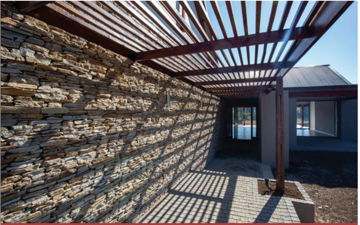
The wood for the pergolas was supplied by Hardwood Lumber with installation by Tholokule Sundecks
